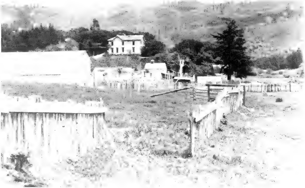
FIGURE 13. Fence offset 8.5 feet. Trace of fault barely visible, running from lower right to upper left through offset. Photograph by G.K. Gilbert. (G.K. Gilbert Collection [N7583-C], California Academy of Sciences Archives.) (Also in Gilbert 1907b, pl. 1, fig. B.)
